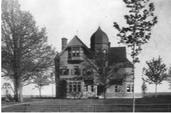
Figure 1 D.R. and Helen Noyes home at 366 Summit, where the first NSCDA-MN meeting was held. It was demolished in 1925.
